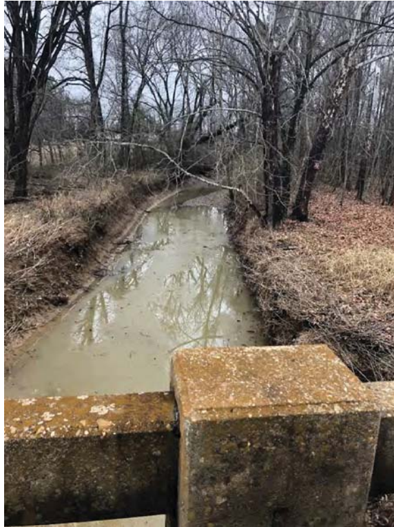
Downstream From Bridge
