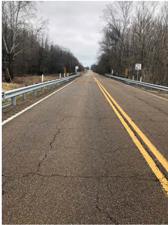
Eastbound Approach of Bridge
