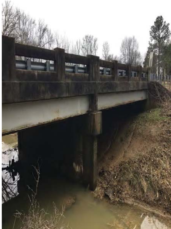
Outlet Pier from East Bank
